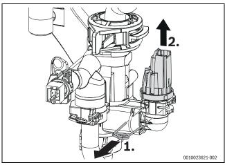
Fig. 105 Removing pressure sensor
