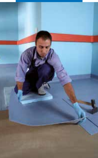
Installing PVC floor tiles
